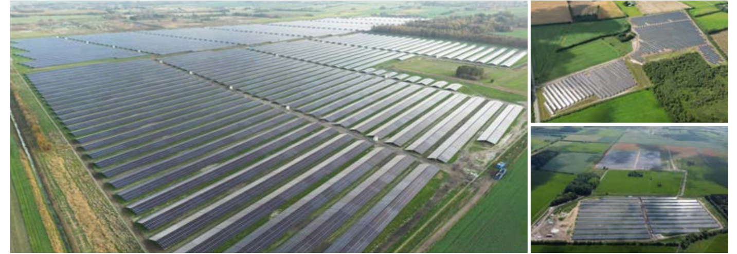
Denmark Projects | 328.00 MWp
