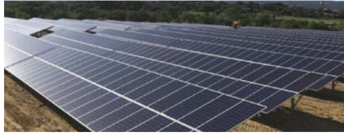
45.60 MWp Type: Ground Mounted Year: 2022 Location: Poland Status: Under Construction
