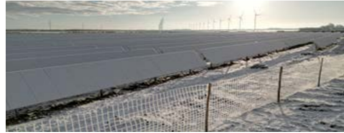
29.00 MWp Type: Ground Mounted Year: 2022 Location: Denmark Status: Under Construction
