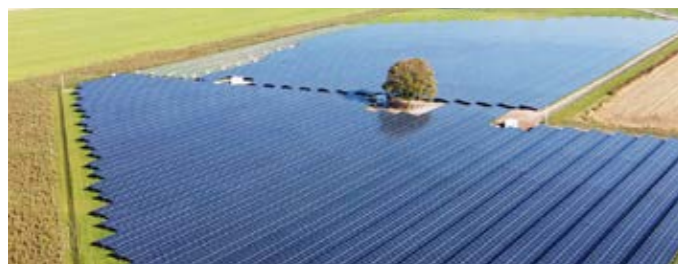
19.00 MWp Type: Ground Mounted Year: 2021 Location: The Netherlands Status: Completed
