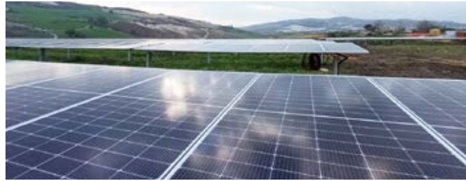
17.00 MWp Type: Ground Mounted Year: 2022 Location: Italy Status: Under Construction
