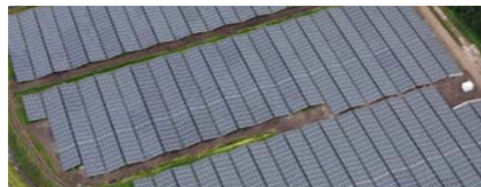
18.00 MWp Type: Ground Mounted Year: 2021 Location: The Netherlands Status: Completed
