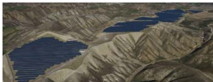
14.00 MWp Type: Ground Mounted Year: 2017 Location: Turkey Status: Completed
